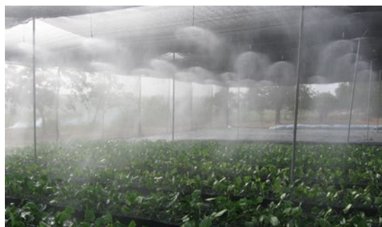
Simple humidification system
