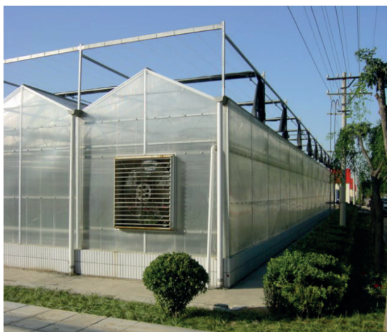
Pad/fan system and a movable outdoor screen
